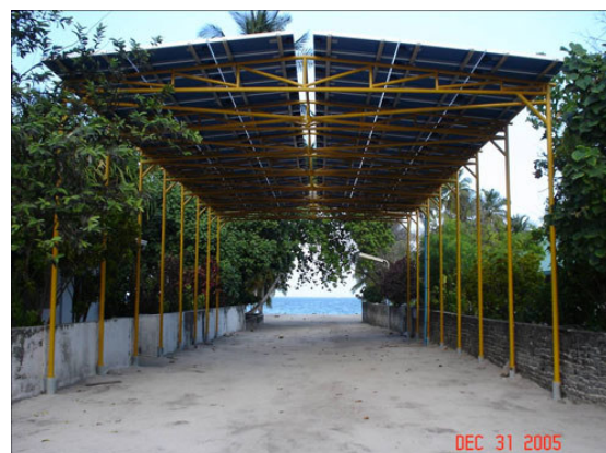
Figure 6: PV system at Mandhoo
