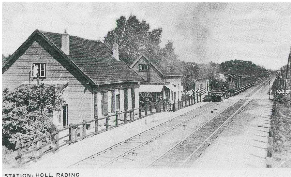
STATION. HOLL. RADING
