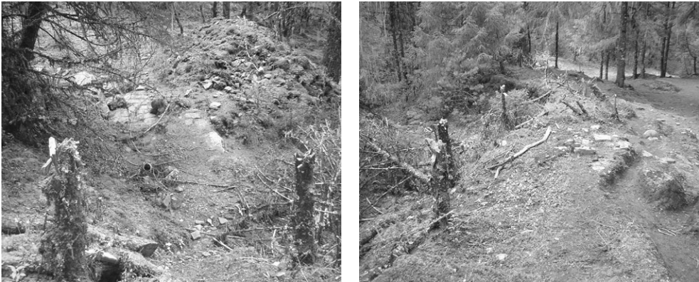
Figure 5.5a and 5.5b Erosion on the Druk Path: The picture left shows the traditional stone paved path, not being used anymore, while the picture right shows the alternative route taken by large groups of horsemen just a few meters to right (the cut down tree is the same one) (Pictures by Vermeulen, 2005)
