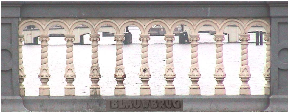
Figure 2 Torsade: Rope molding, cable molding. A Norman molding enrichment like a twisted rope; any ornamental twist [17]. Example: Blauwbrug, Amsterdam
