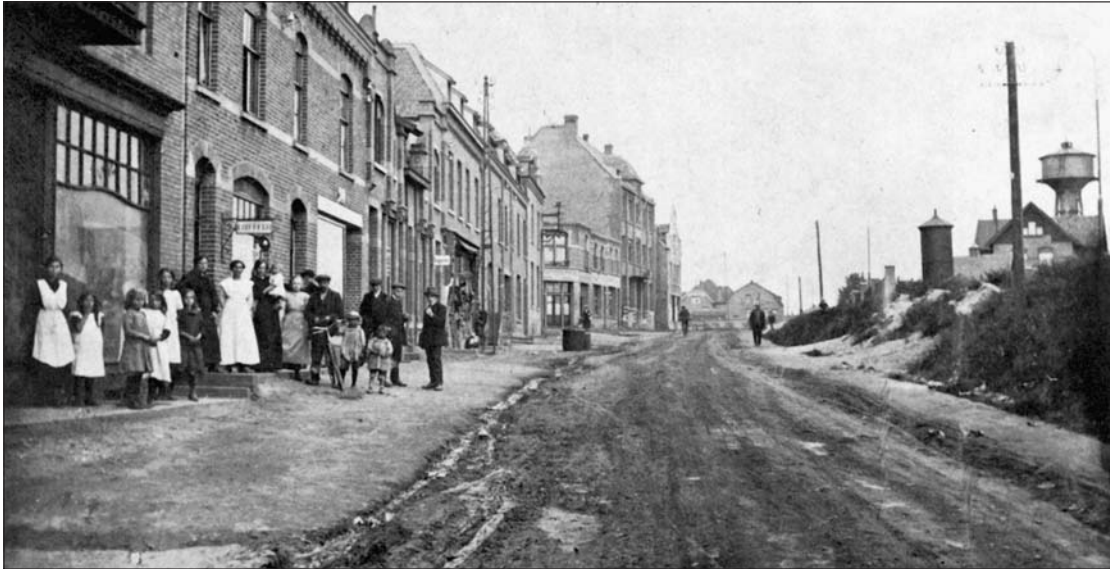
Fig. 2. Akerstraat ca. 1919. Luxor theatre, built in the summer of 1919, was located on the main road. The road is not metalled indicating that the town was still developing. On the right, the mine buildings are visible. [Courtesy Gemeentearchief Heerlen.]
