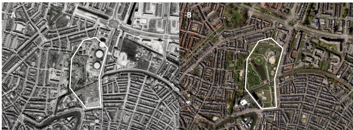
Figure 1. Aerial view of the Griffpark in 1967 (panel A) and 2018 (panel B). The white outline indicates the area that is isolated by the underground bentonite wall.
