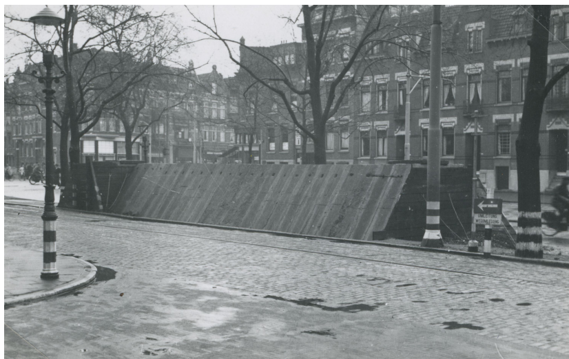
Figure 1 Corridor shelter, Henegouwerlaan, Rotterdam (Beeldbank WO2 – Verzetsmuseum, Amsterdam, reproduced with permission)
