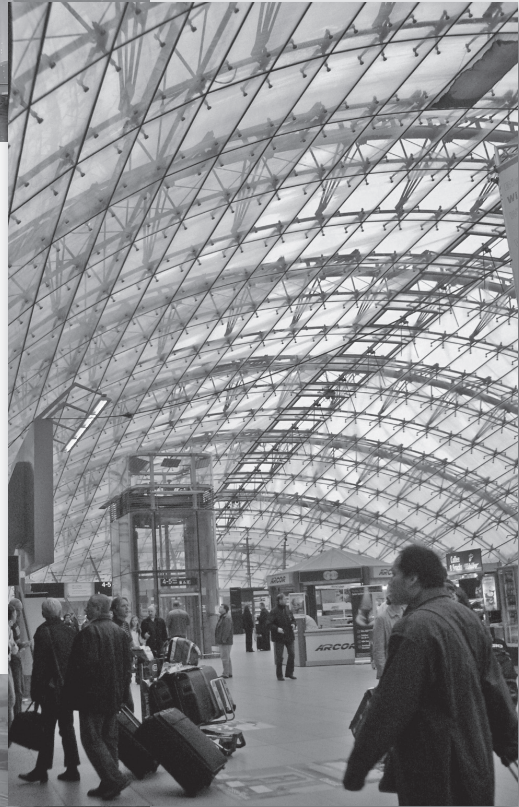
AIRRAIL Center inside
