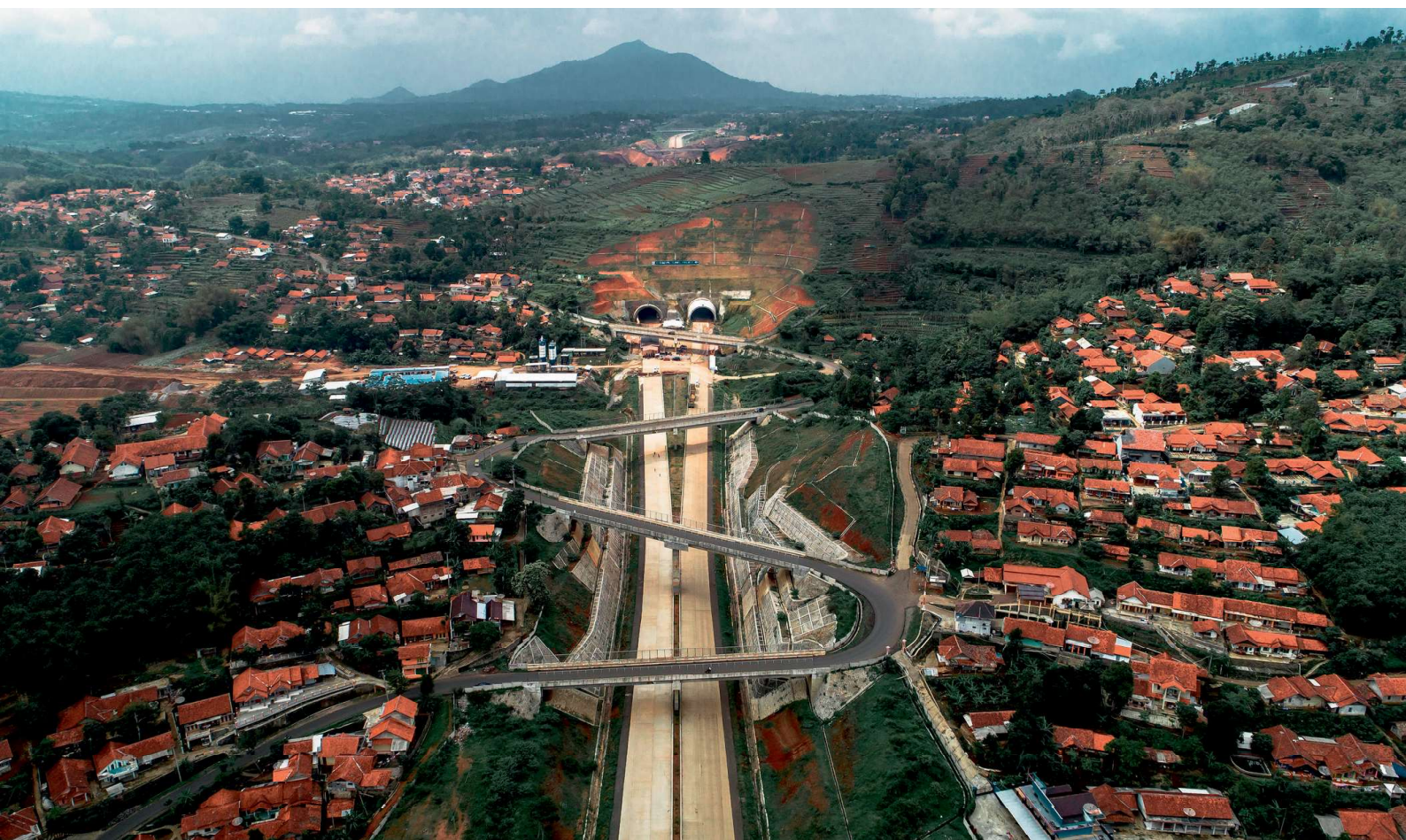
Cisumdawu highway and tunnel, Sumedang, Indonesia ©Klasikdisko
