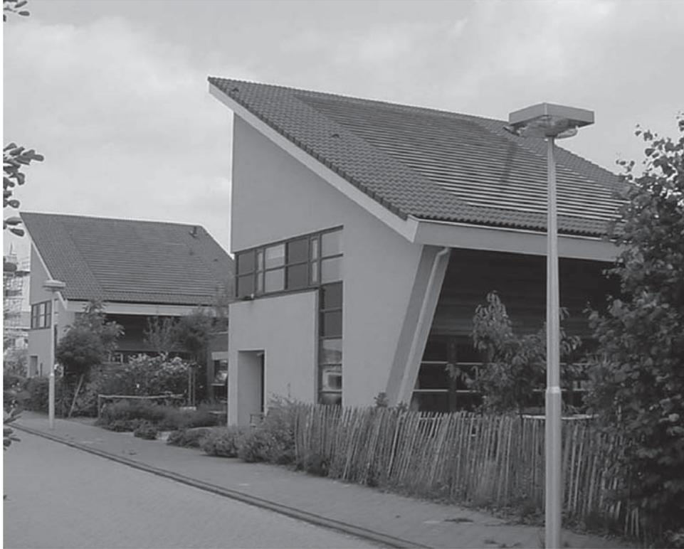
*5.2 The Information Centre for Sustainable Living in Utrecht, the Netherlands. It was built as a 'zero-energy house' with 50 m<sup>2</sup> of photovoltaic panels integrated in the roof and high isolation levels (roof and façades 6 m<sup>2</sup>.K/W; floor 5 m<sup>2</sup>.K/W; triple windows 0.7 W/m<sup>2</sup>.K). It is intended to have a modern, non-alternative look. (For more information see *Duurzaam Huis 2004*.)*
