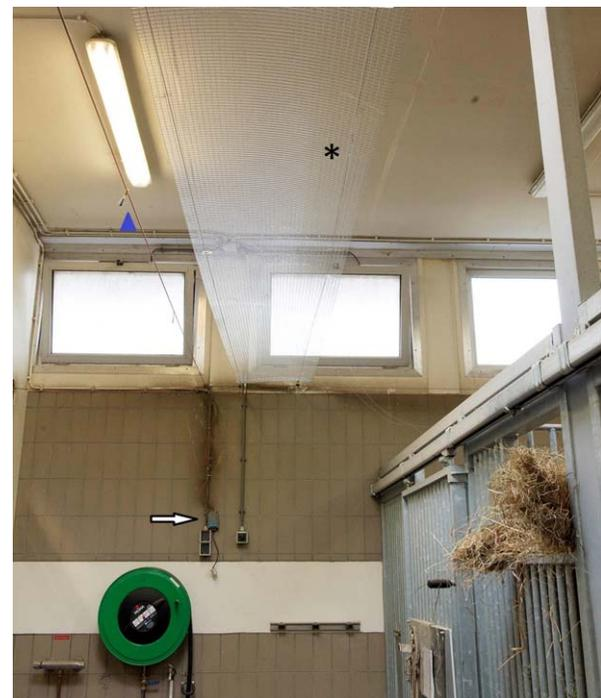
**FIGURE 2** Pictures of the ionization installation in 1 of the units (high dust unit using straw as bedding and dry hay as roughage), showing the ionization device (arrow), corona wires (arrowhead) and iron wires with additional mesh (\*)
