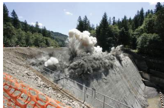
Figure 18. Demolition of Marmot Dam in 2007 (Keller, 2010)
