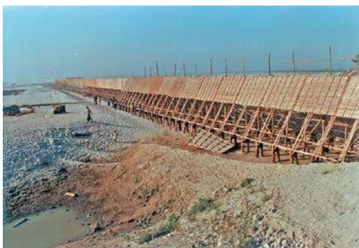
Figure 22: Bandals used to close a secondary channel (Mosselman, 2006)
