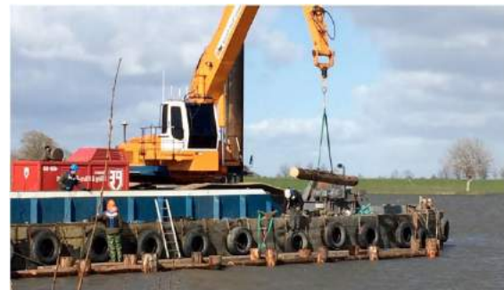
Figure 2. Construction of the screen.
