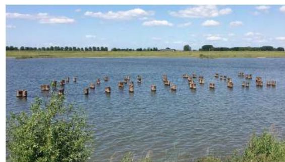
Figure 3. The wooden screen in the river.
