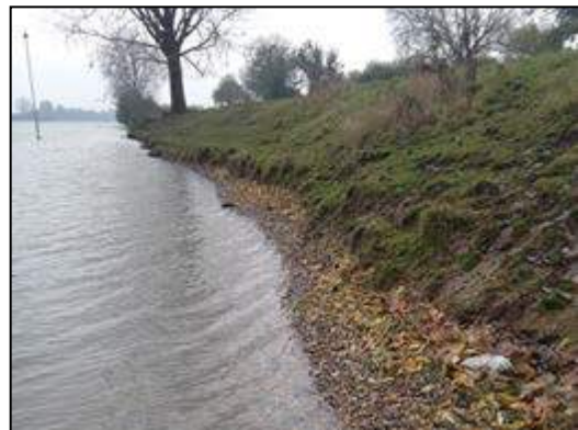
Figure 1. Uniform erosion pattern characterized by short grass-covered banks with gravel at the toe.
