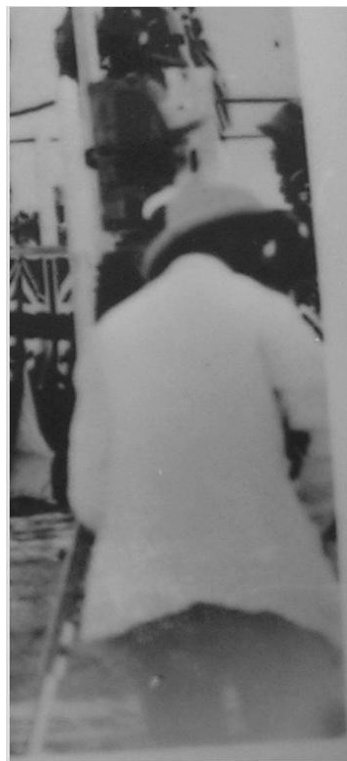
Fig. 11. Detail. Note the rectangular box of the camera (beyond his hat), and the leg of the tripod to his left.
